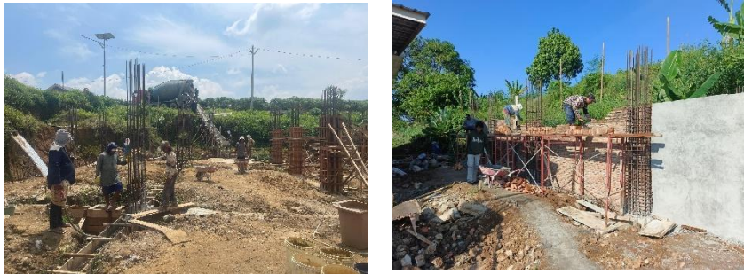
Figure 4. Implementation of the Construction of the Quasi-Holy Cross Catholic Church Tj. Anom
